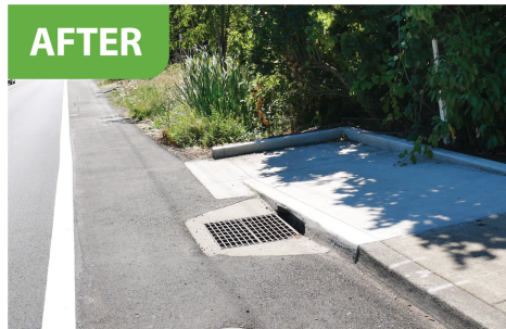
End of the sidewalk near the intersection of SW Hall Boulevard and SW 92nd Avenue before and after ADA compliant upgrades and stormwater drainage upgrades .
