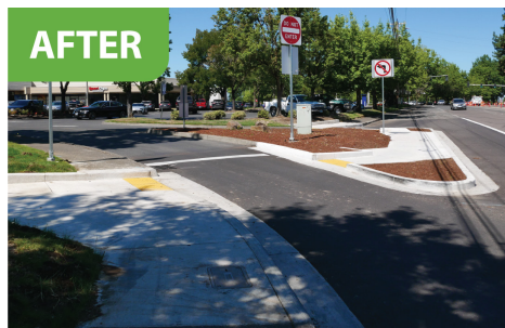
Sidewalk curb ramps at an existing driveway before and after ADA compliant sidewalk curb ramp upgrades .
